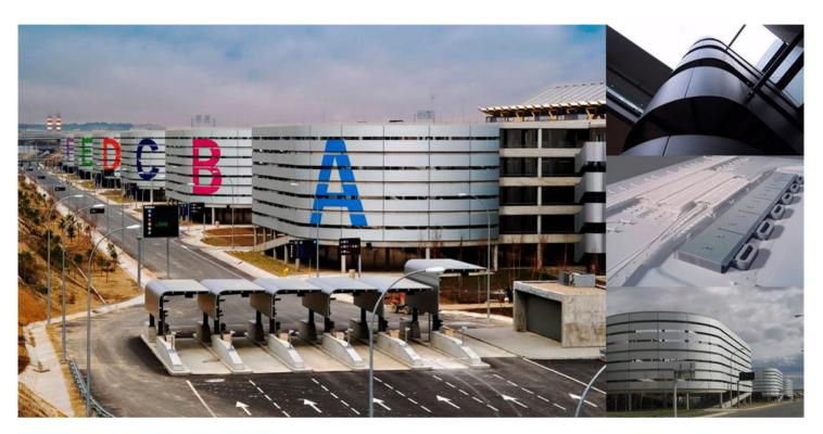
The car park building of the new terminal of Barajas Airport, of  $656,40 \times 80,00 \text{ m}$  on plan and six levels, is divided into six modules of  $112,00 \times 80,00 \text{ m}$ , without joints. Structurally, it is a 0,38 m deep reinforced concrete waffle slab, supported by a grid of columns of  $8,00 \times 8,00 \text{ m}$ .
